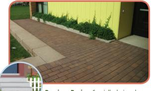
**Pervious Paving:** Specially designed paving stones, bricks, or pavers that allow water to soak into the ground below.
