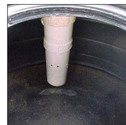
The interior view of a septic tank.
