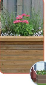
**Downspout Planter:** Connected to the roof downspout, these planters slow water down before entering the sewer while irrigating plants and
