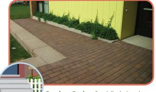
**Pervious Paving:** Specially designed paving stones, bricks, or pavers that allow water to soak into the ground below.
