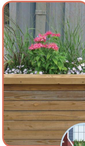
**Downspout Planter:** Connected to the roof downspout, these planters slow water down before entering the sewer while irrigating plants and removing pollutants.
